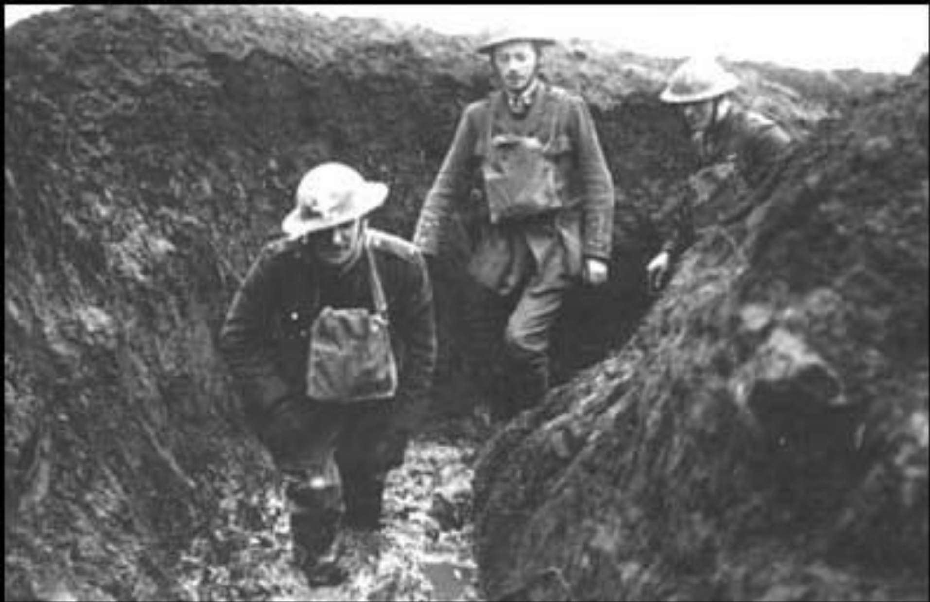
Officers walking through a flooded communication trench.
