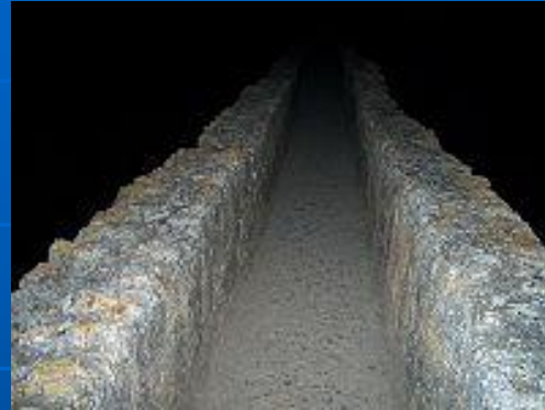
The water-carrying channel of the Aqueduct
